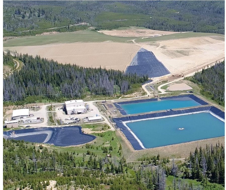
Beartrack Plant Site
